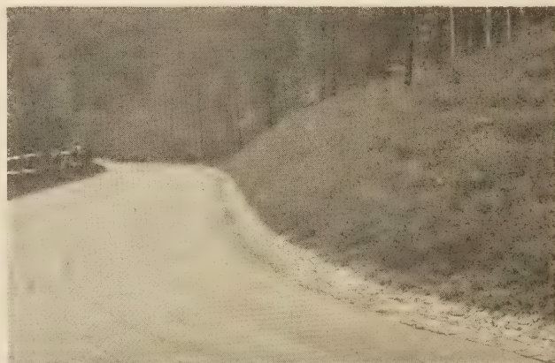
SLOPES COVERED WITH DESIRABLE VEGETATION MAKE THE ROADSIDES ATTRACTIVE AND REDUCE MAINTENANCE COSTS.
